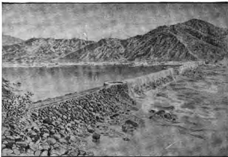
FIG. 195.—View of San Fernando Submerged Dam.
